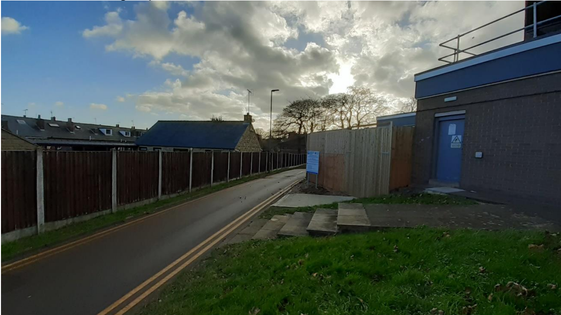
Figure 3 1Gosber Street is located to the east
