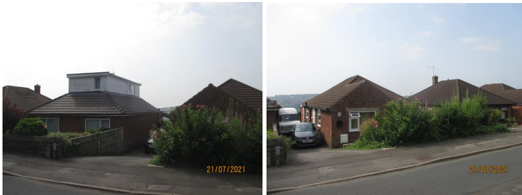
Figure 2: Photo taken from Bents Crescent
