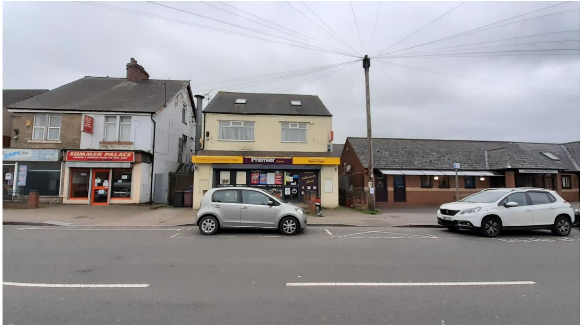
Figure 2 205-207 Sheffield Road as existing showing narrow access rear on left of the building
