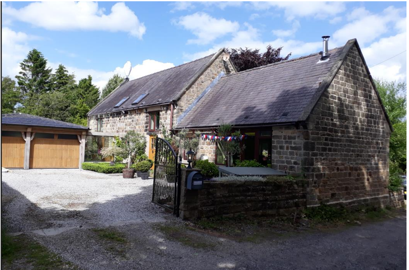
Fig 1 – south and west elevations
